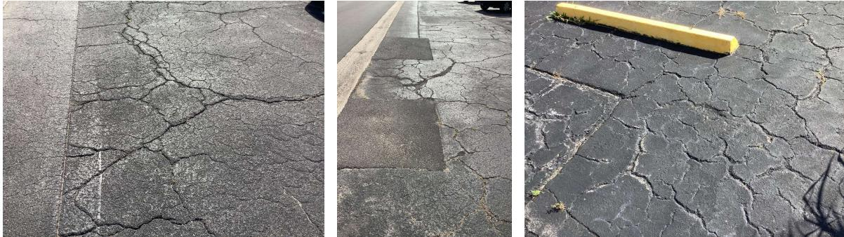
This category refers to costs associated with the seal coating of asphalt parking areas. Barring unforeseen damage, and assuming proper and routine maintenance, a minimum useful life of approximately 5-7 years can be expected. The current replacement cost estimate is based on industry standards, national cost estimating indexes, and our experience with this type of component.
