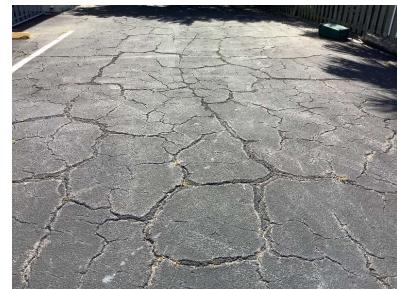
This category refers to costs associated with the milling, recoating, and striping of asphalt parking areas. Barring unforeseen damage, and assuming proper and routine maintenance, a minimum useful life of approximately 20 years can be expected. The current replacement cost estimate is based on industry standards, national cost estimating indexes, and our experience with this type of component.
